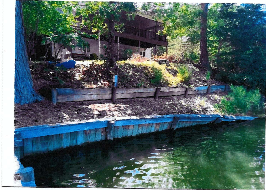
815 river view dr kinsale va (bulkhead repair)
